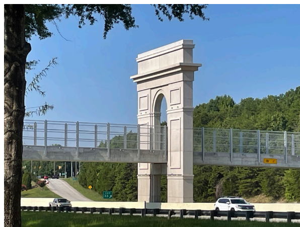
New pedestrian/bike bridge over I-385
