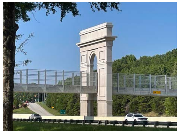
New pedestrian/bike bridge over I-385
