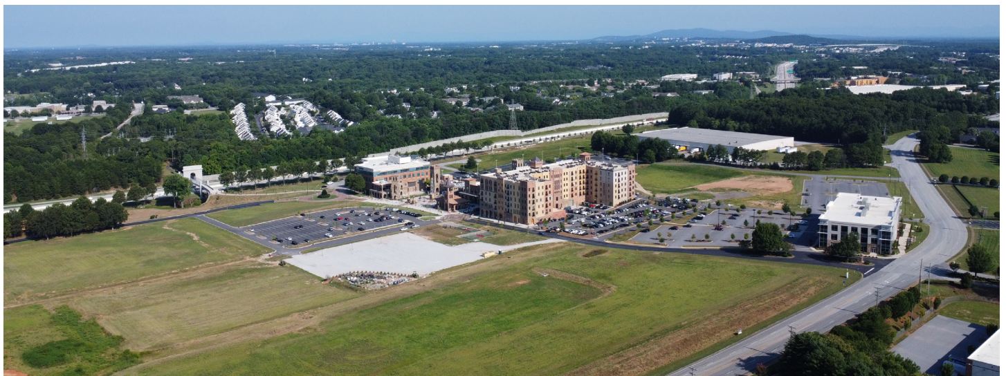
View of BridgeWay Station (Phase One) along I-385
