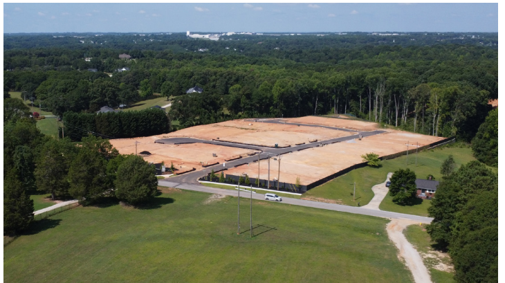
Neighborhood Construction near Sunset Park (Fowler Circle)
