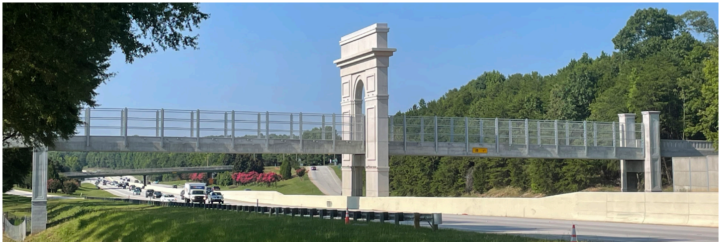
I-385 Pedestrian and Bicycle Bridge - Future Swamp Rabbit Trail Connection to BridgeWay
