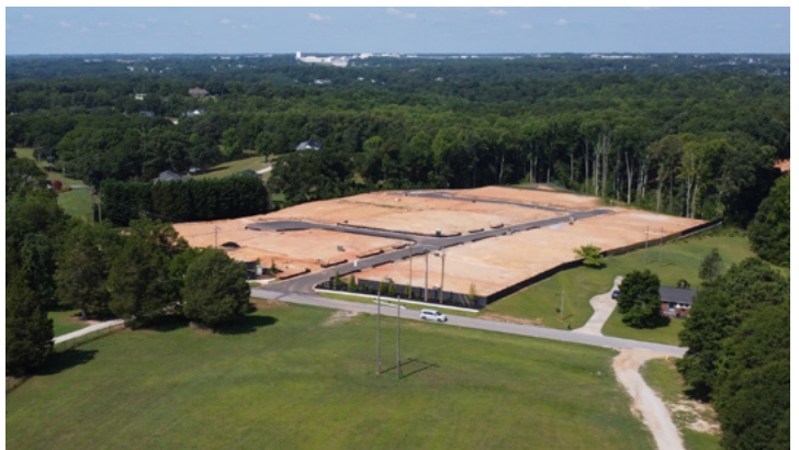
Neighborhood Construction near Sunset Park (Fowler Circle)
