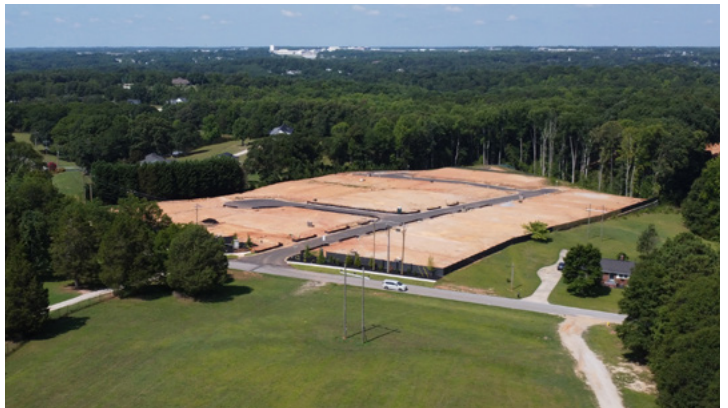
Neighborhood Construction near Sunset Park (Fowler Circle)
